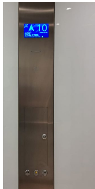
COP with hidden mechanical button panel
